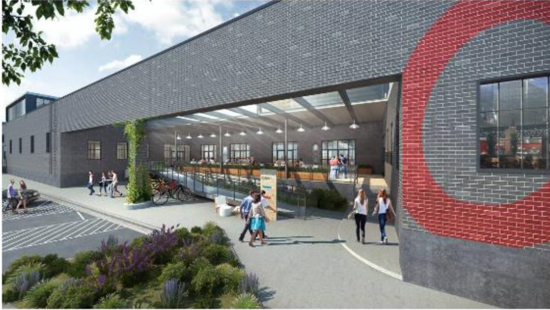
Rendering of the Gama Goat building at Camp North End. Courtesy ATCO
